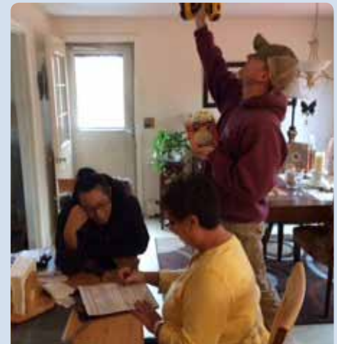
Pictured left to right is Allyssa Hathaway, MWT emergency preparedness specialist; Nancy Martin, MWT clerk; and Travis Melick, MWT emergency preparedness intern installing new detectors.
